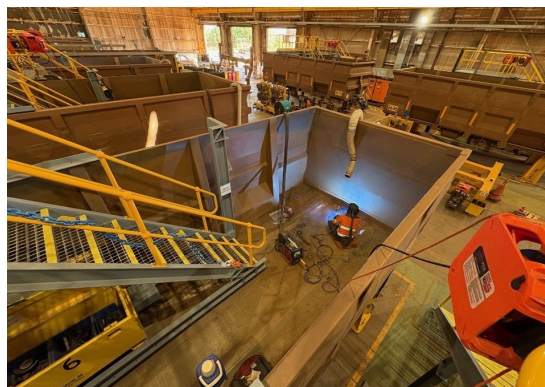
INTERNAL WAGON REPAIR AT THE WORKFACE
